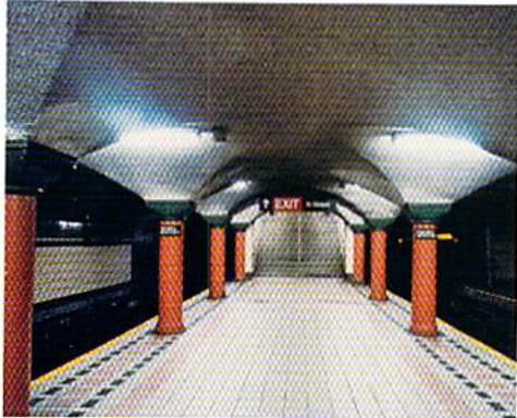
PATH System Pavonia/ Newport Station Port Authority of New York and New Jersey
